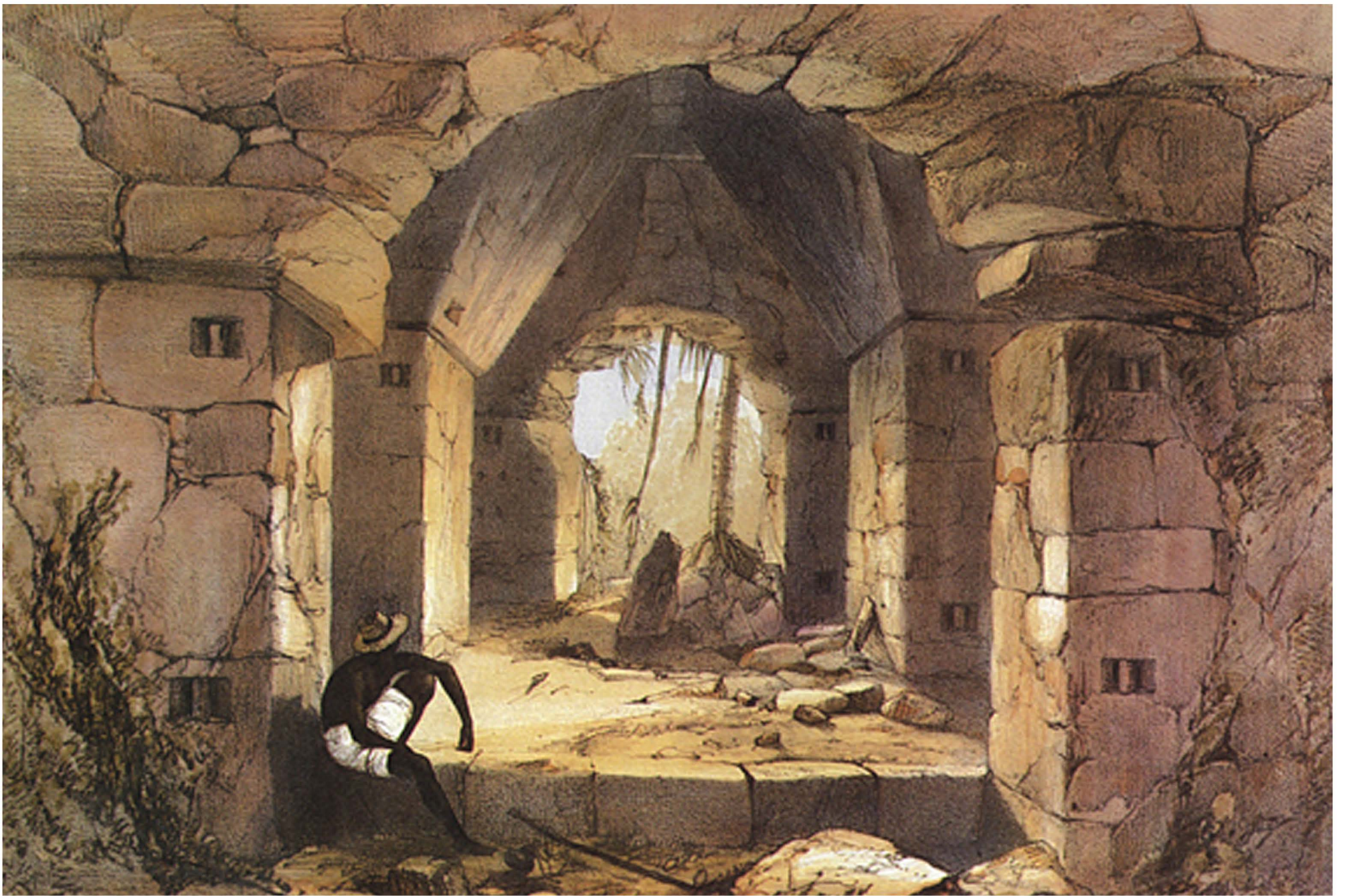
Interior of Casa III Palenque
